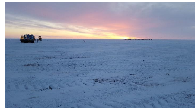
Snow pre-packing activities prior to ice-road construction
